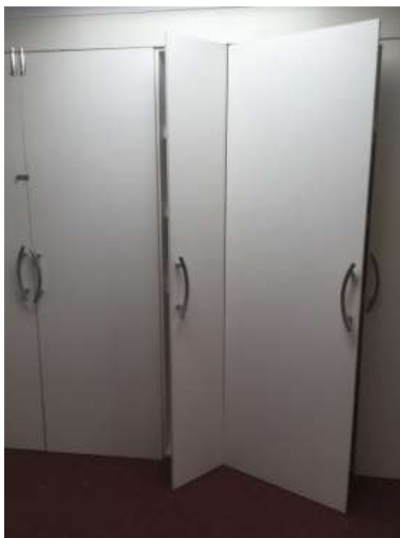
2no double doors each 675x2125 and 1no 340x2125
